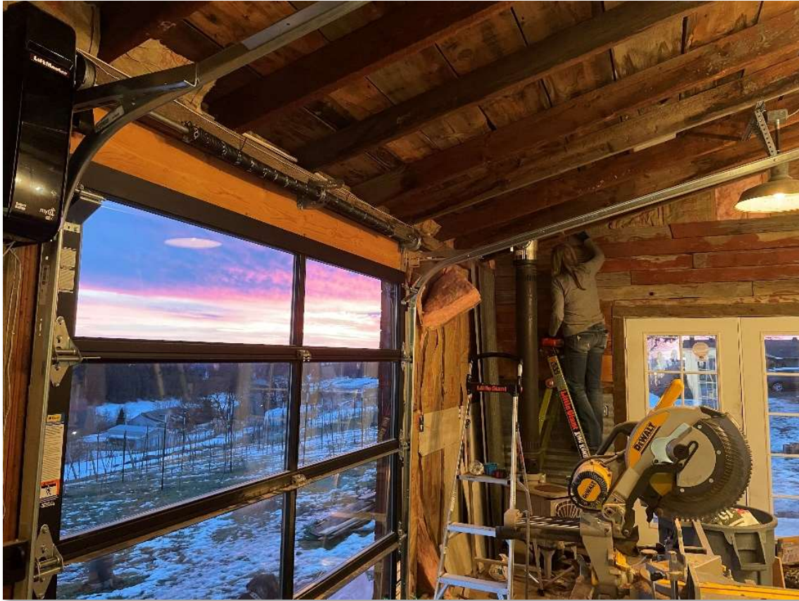
Interior Finishing - winter of '21/'22
