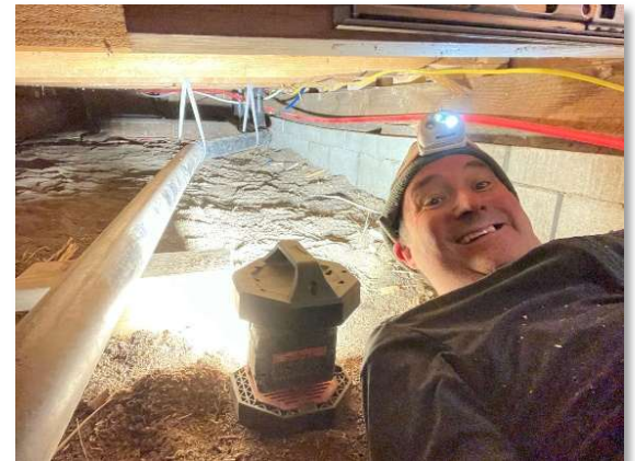
plumbing under the bunkhouse
